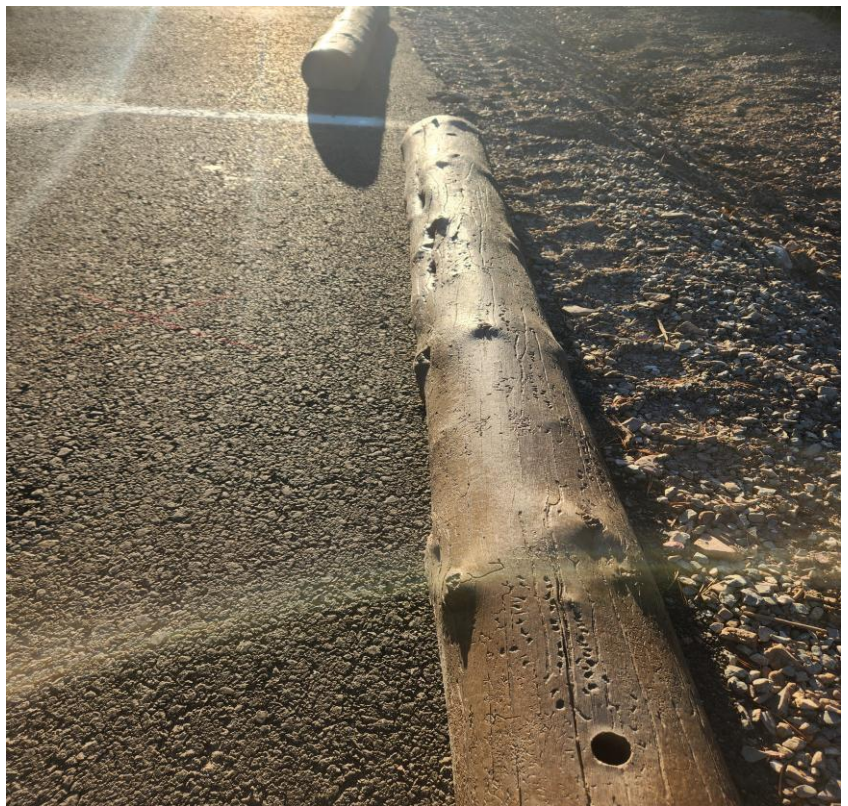
Precast concrete wheelstop
