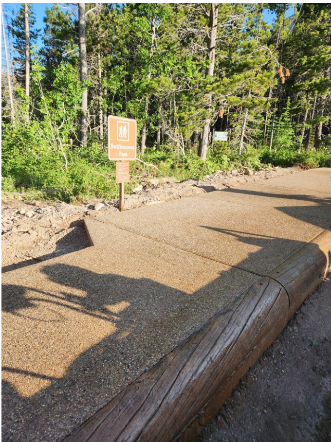
Concrete log curb set on sight with exposed aggregate sidewalk.
